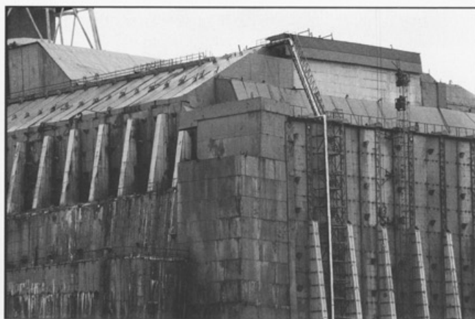
James Lerager, The Chernobyl Sarcophagus . The Chernobyl Sarcophagus, built with the labor of 600,000 people and originally intended to stand for decades, was already buckling and disintegrating within a few years after construction was completed in 1987. Now in danger of collapsing, it is to be superseded by a much larger structure—arching over the entire reactor building and original sarcophagus—to be constructed by an international consortium at a cost currently estimated at $800 million. Inside the cracking building still contains large quantities of the reactor's radioactive materials. Robotic remote control and automated equipment, designed to monitor conditions inside the sarcophagus, has broken down under intense radiation.
